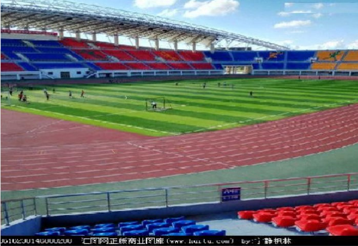
Semi-open stadium sound reinforcement
