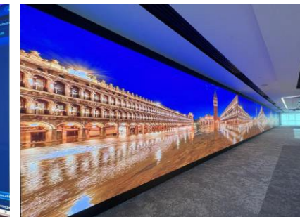
Transco command center in Abu Dhabi, UAE
